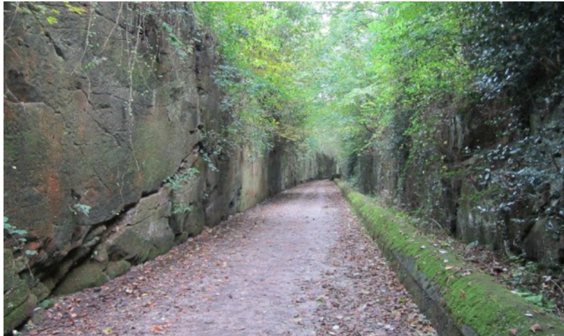
Photo taken at Neston railway cutting on the former Hooton to West Kirby railway line.. Creative Commons Attribution-Share Alike 3.0 Unported
