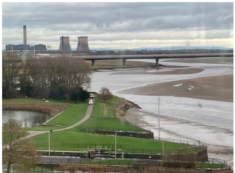
Fiddlers Ferry Power Station from the Observatory Tower
